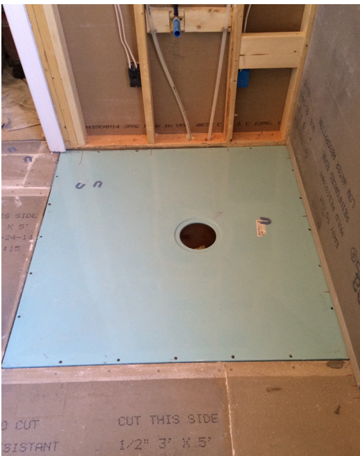
Classic shower base installed on joists.
